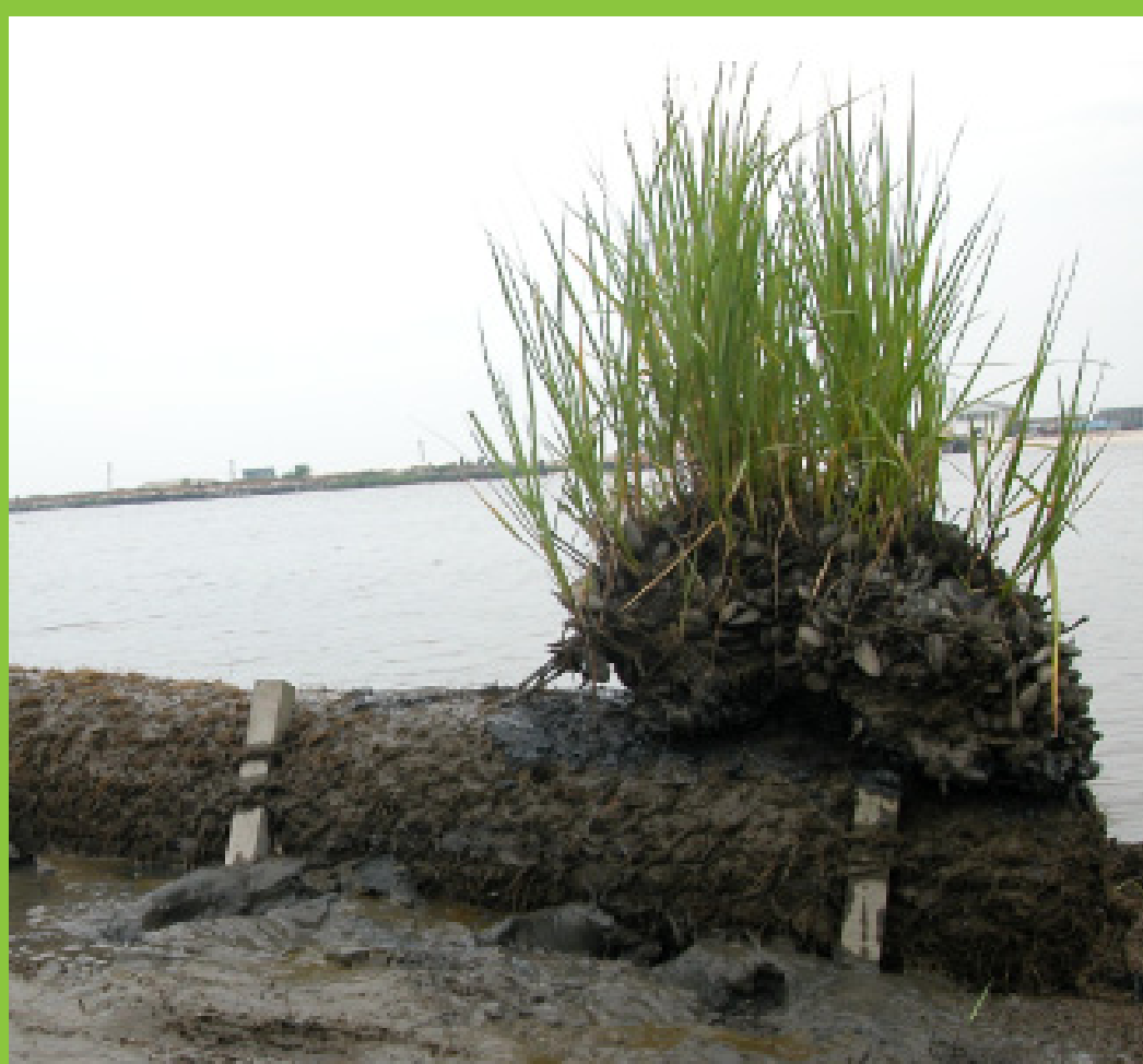
Figures 20. A salvaged plug from the nearby area on a coir log. Note the large established root mass around the plants embedded with mussels.
