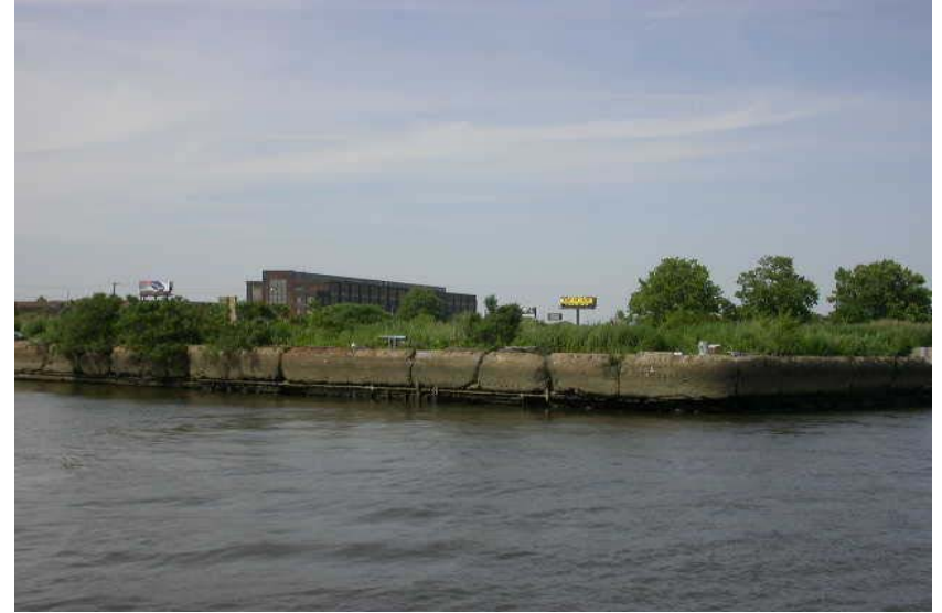
Failing Bulkheads at Old Phila. Piers
