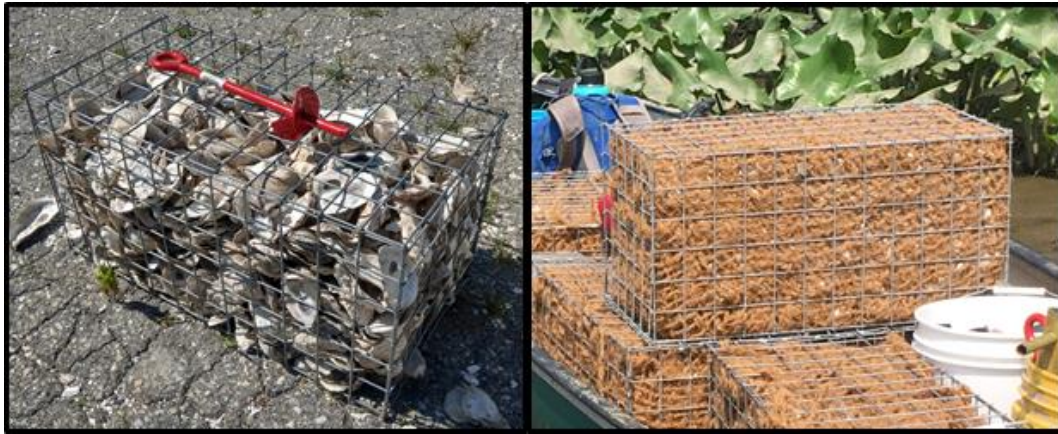
Figure 3. Gabions filled with oyster shell (left) and additional coir liner (right).
